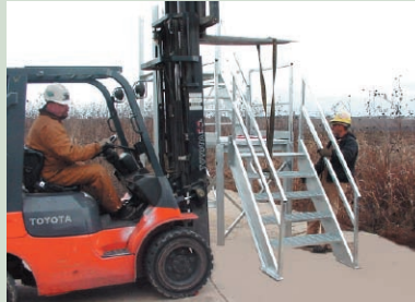
Step 9: Lower Stairs to WashDown Module
